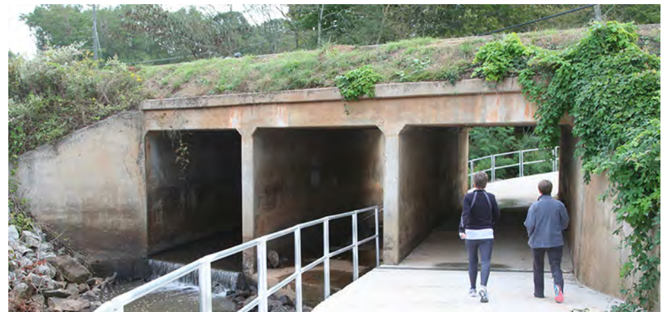
Multi-use trail through existing box culvert requires a 7'6" minimum vertical clearance.
